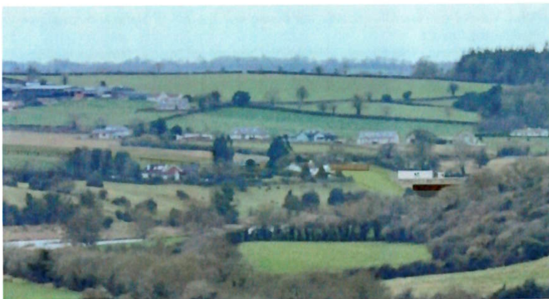
Detail of VPT 01, focussing in on the southern approach to the proposed new Boyne Bridge and what appears to be the Rossnaree overbridge: Year 1
