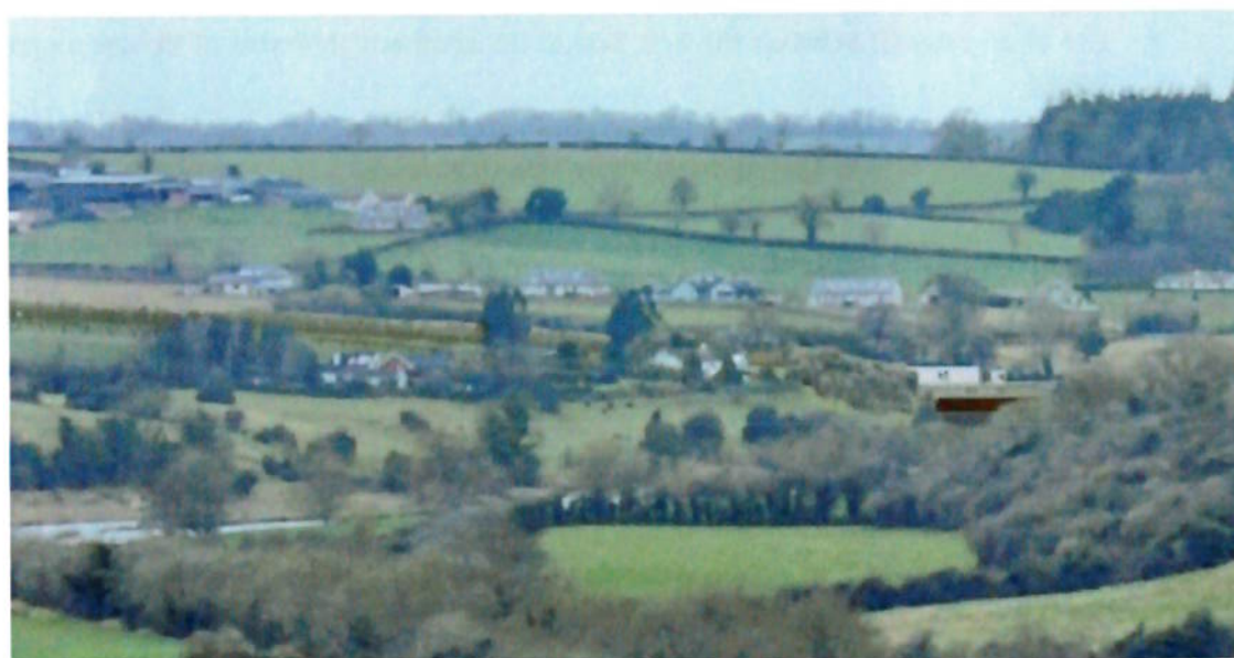
Detail of VPT 01, focussing in on the southern approach to the proposed new Boyne Bridge and the Rossnaree overbridge: Year 10
